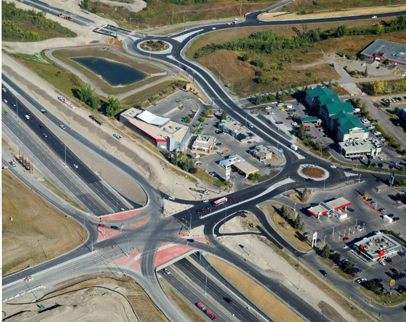
Trans-Canada Highway/Bowfort Road Interchange Calgary, Alberta
